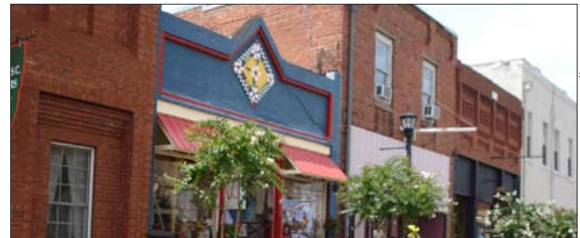
Creative Primary sign used in sign band area and coordinated with the overall facade color scheme.
