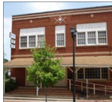
A typical 2-story historic commercial building in Dallas.
