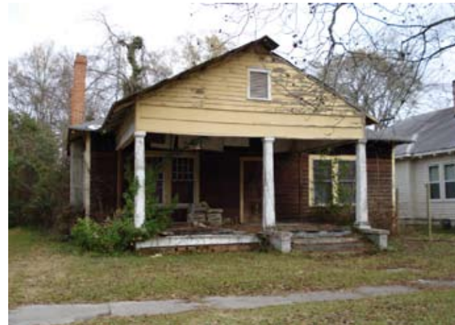
Fig. 7.1: Stabilization Measures for Vacant Property
